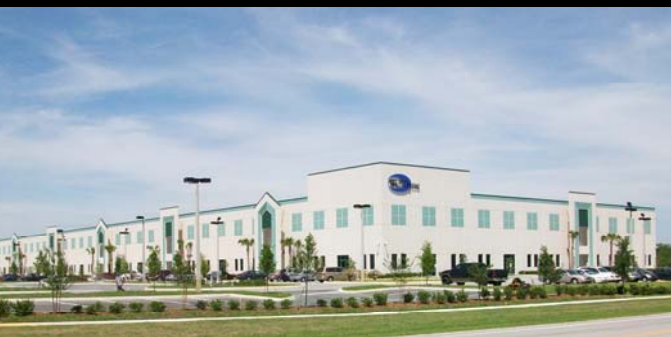
WellDyneRx Southeastern Operations
