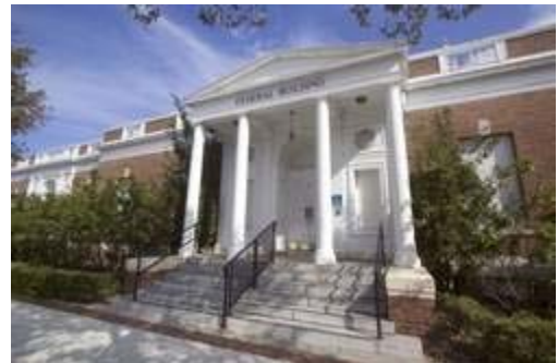
MICHAEL WILSON | THE LEDGER The old Federal Building at the corner of South Tennessee Avenue and East Lemon Street in downtown Lakeland. November 19, 2009.
