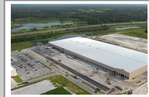
FIRST INDUSTRIAL'S 400,000 SQ. FT. SPEC BUILDING AT FIRSTPARK@BRIDGEWATER IN LAKELAND. USER HOME DEPOT SUPPLY IS TAKING 240,000 SQ. FT.
